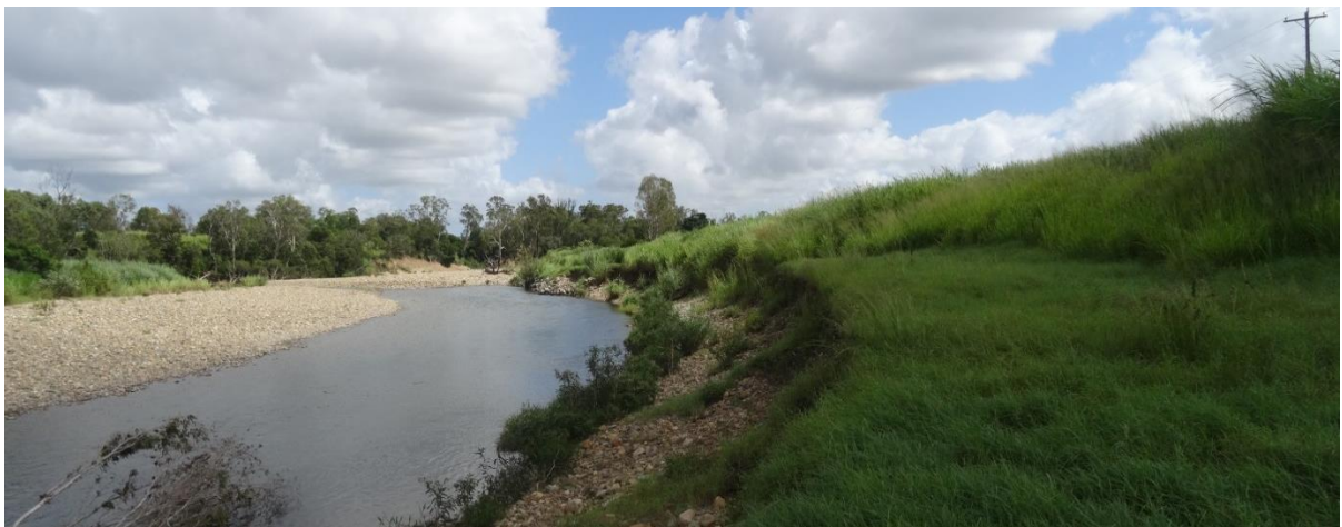
Figure 109. Looking downstream along the right bank located 1.5 km upstream of the Boundary Creek confluence. Site is subject to meander migration.
