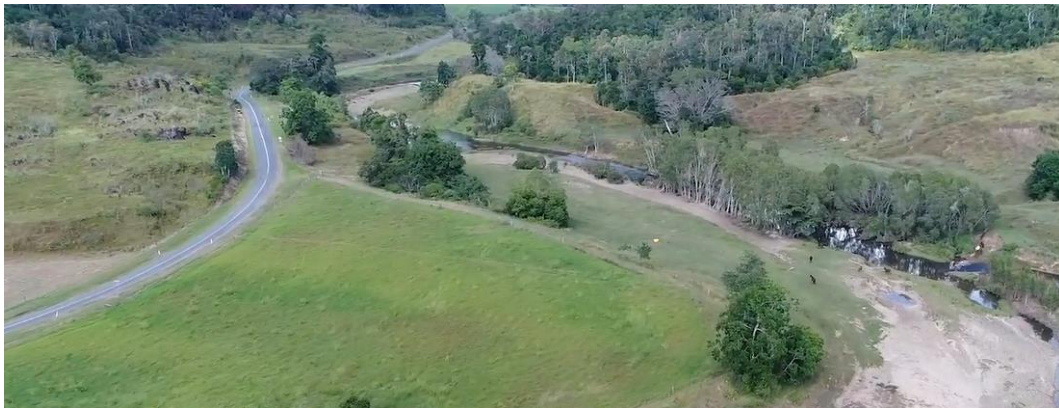
Figure 83. Murray Creek through the bedrock-controlled section upstream of the Bruce Highway.
