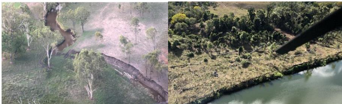
Figure 2: Stream bank erosion along the Mimosa Creek (Dawson River catchment) (left) and Burnett River (right)
