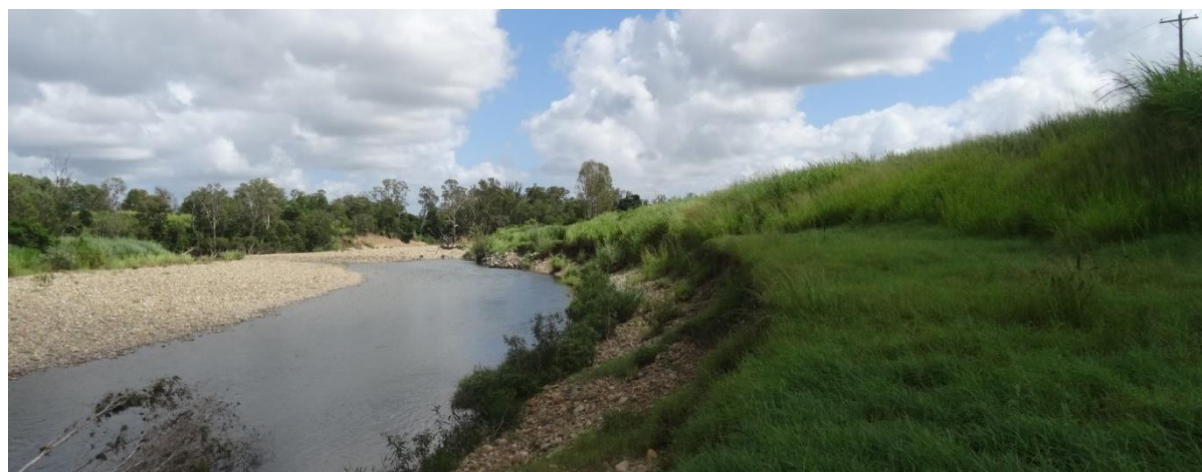
Figure 78: Looking downstream along the right bank located 1.5 km upstream of the Boundary Creek confluence. Site is subject to meander migration
