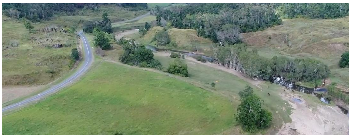
Figure 65: Murray Creek through the bedrock-controlled section upstream of the Bruce Highway
