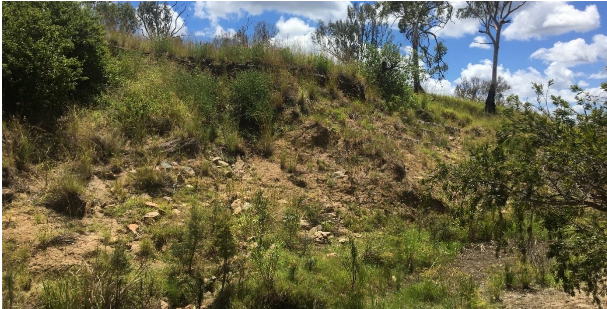
Figure 33: An example of a steep and eroding bank in Raglan Creek
