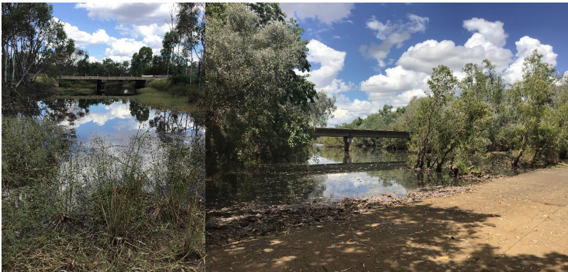
Figure 28. Examples of pooling behind old road crossings in tributaries of the Little River.
