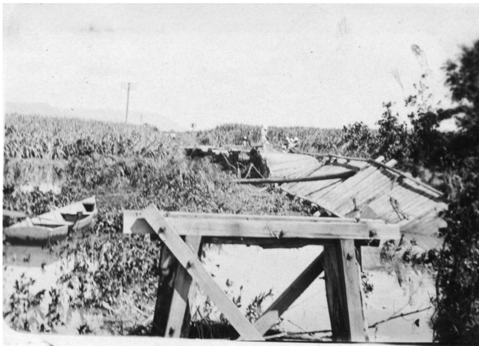
Figure 16: The Stratford bridge over the Barron River, damaged in the 1932 flood (Cairns Historical Society P18037).
