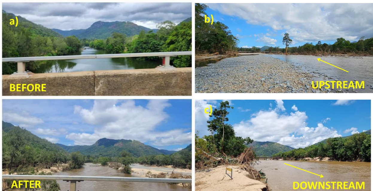
Figure 19: Changes to the Barron River at Caravonica/Kamerunga due to the 17 December 2023 ex-TC Jasper flood, a) the Barron River before and after the flood (photo source: Facebook user upload) and widening of the Barron River b) upstream and c) downstream of the Kamerunga Bridge. The yellow arrow shows the direction of river flow.
